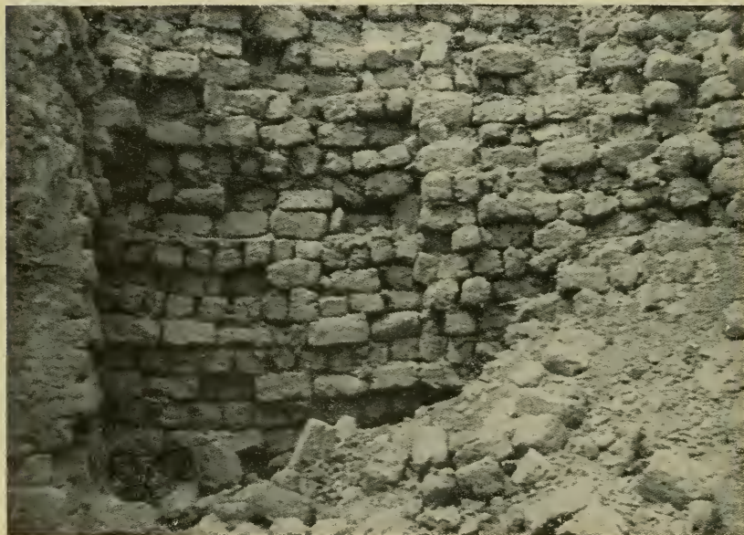
PLATE 16.—Andean masonry types. Top : Pirca construction of the Highlands. Bottom : Packed rectangular adobes of the Coast. (After Means, 1931, fig. 138, from W. V. Alford; and courtesy American Museum of Natural History.)
